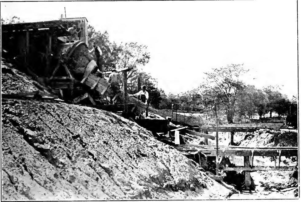
BUILDING THE HARLEM CREEK SEWER, ST. LOUIS, MO.
